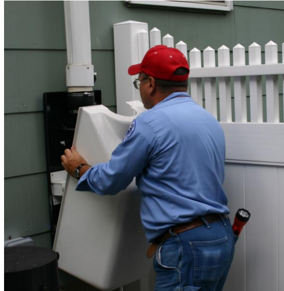
Inspection of SSD fan and weatherproof cover
