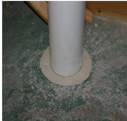
Proper sealing around suction point
